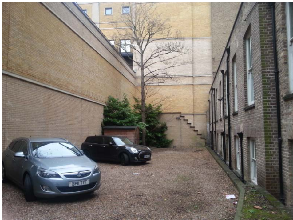
View from Redan Place (top) and eastward view within existing yard area (bottom).
